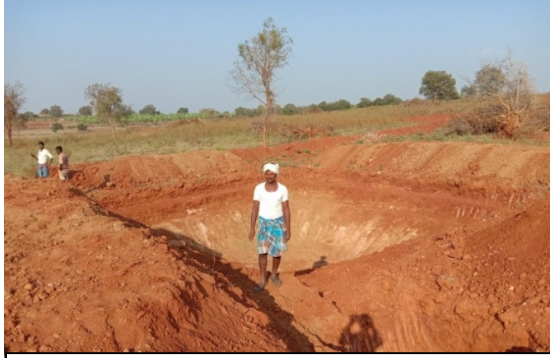
“Construction of Farm Pond in Kudluru”
